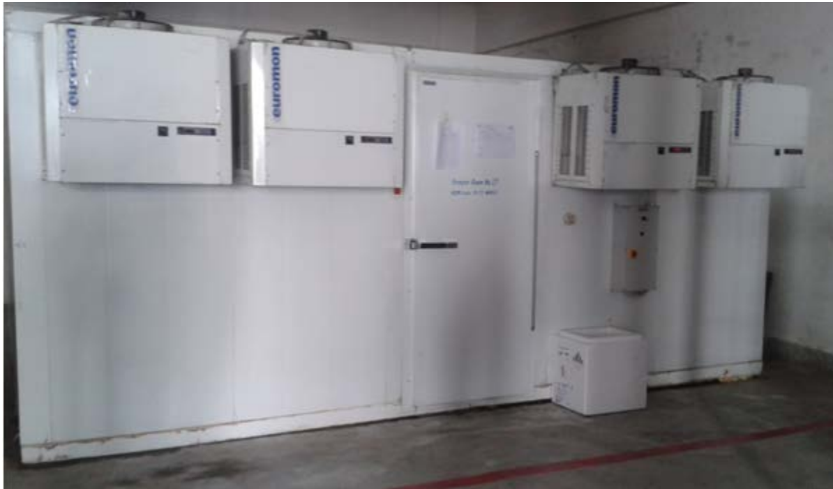
Figure 20. Freezer Room 50 m 3 Capacity at Store
